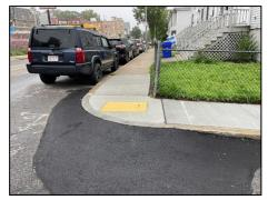
The Federal Highway Administration explains, "[t]here are a number of maintenance, design and pedestrian safety problems with the installation of built-up curb ramps" and that "[t]hey should not be the first choice of curb ramp application." These ramps are unsafe because "[u]sers are more exposed to cars in the roadway" and there is "[n]o clear boundary
