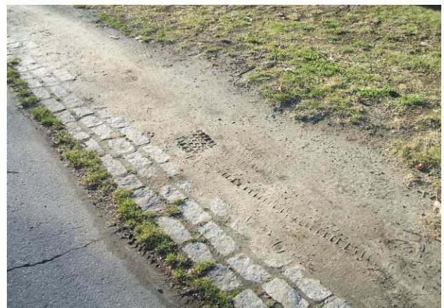
Figure 4. Along Charles St.
