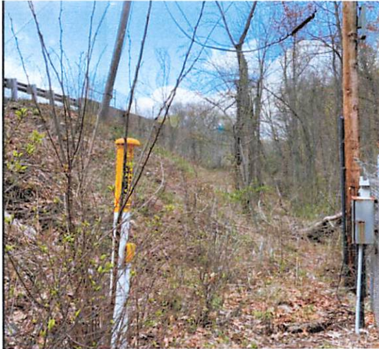
Photo shows the steep slope, TGP pipeline marker and edge of Rt. 2 West.
