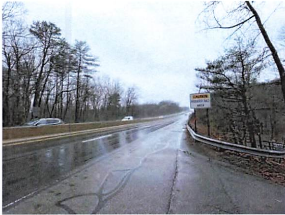
View west along Route 2 at subject
