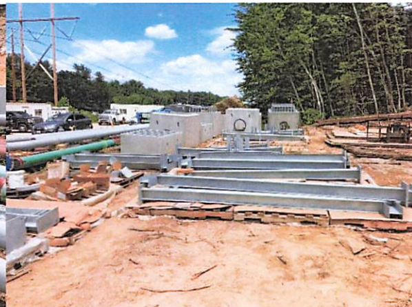
Pipe Supports, prior to install.
