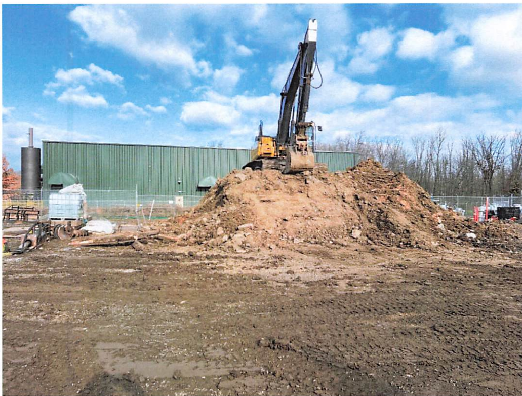
Soil/Equipment, moving soil to allow workable access near pile.
