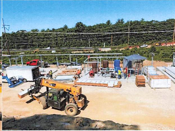
Preparation for stick-built Heater Building Pallets of material starting to arrive.
