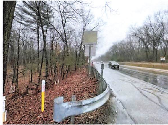
View east along Route 2 at subject
